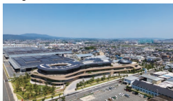
Daiwa House Group MIRAI KACHI KYOSO Center "Kotokurie"
